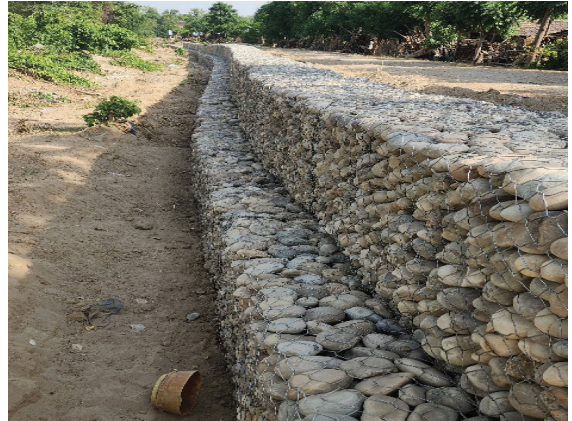
Figure 12 Check dam Installation-Jalandhara CFUG-Dhakeri, Banke
