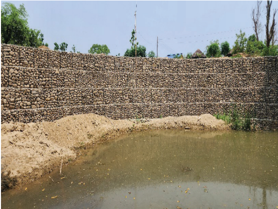
Figure 11 Check dam Installation-Sadabahar CFUG-Mehemenpur, Banke
